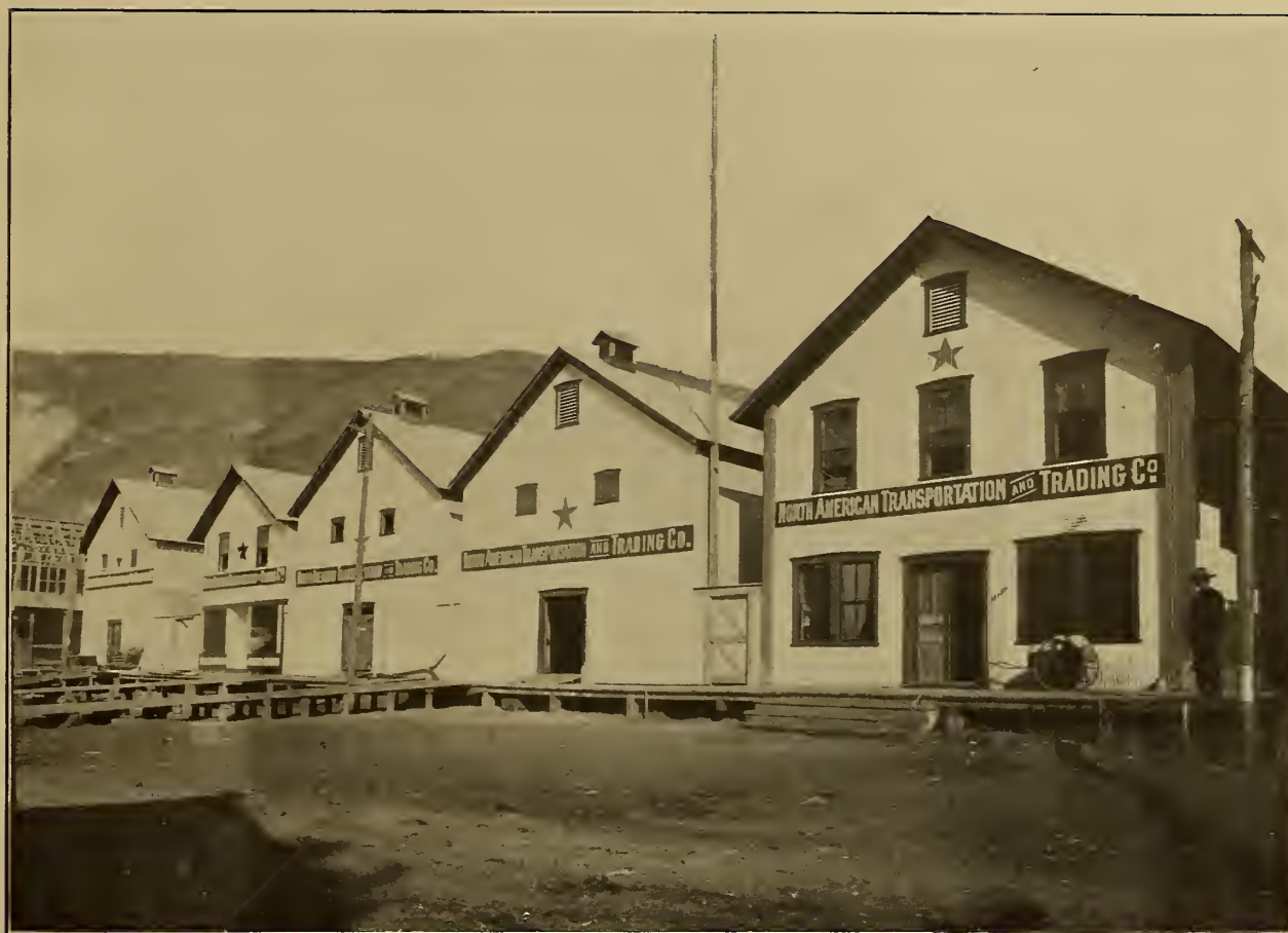
N. A. T. CO.'S OLD STORES AND WAREHOUSES, DAWSON CITY
